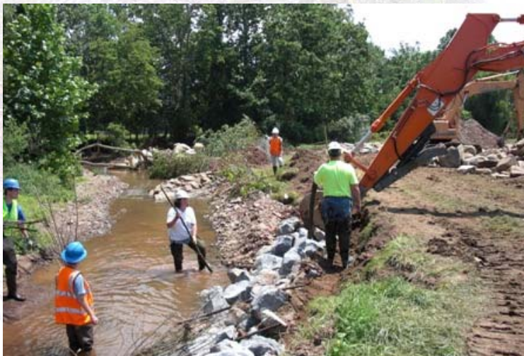
Meander #1 installing LPSTP stone. June 2009
